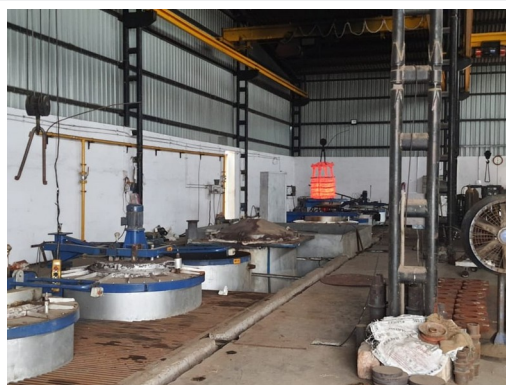
CHARGE UNDER THE CRANE
